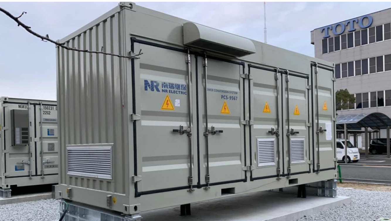
NR supplied PCS and control system for China's first Sodium Sulfur (NaS) BESS
